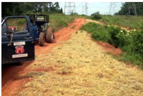
Photo courtesy of ADEQ Streambank Stabilization Plan
