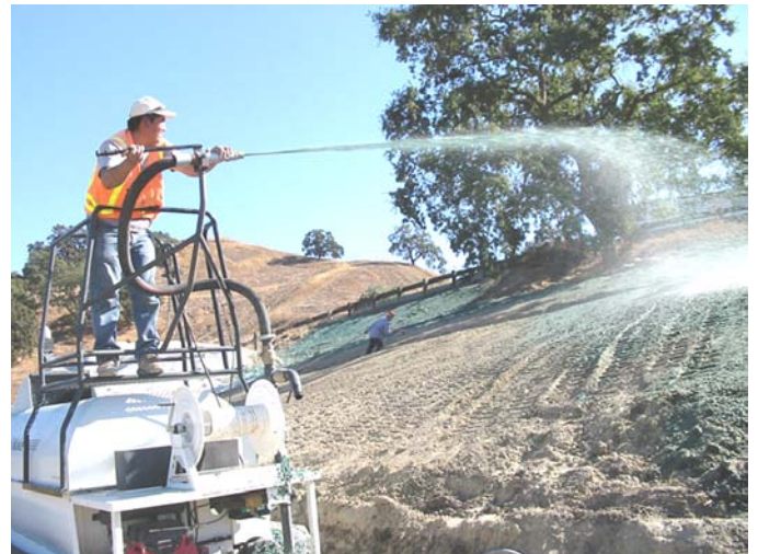
Photo courtesy of ADEQ Streambank Stabilization
