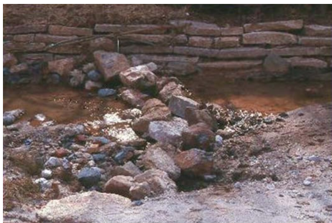
Photo courtesy of ADEQ Streambank Stabilization Plan
