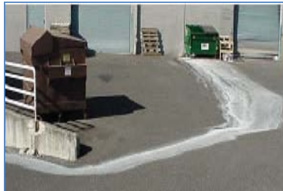
Drainage from industrial dumpster Photo courtesy of ADEQ NPS Program
